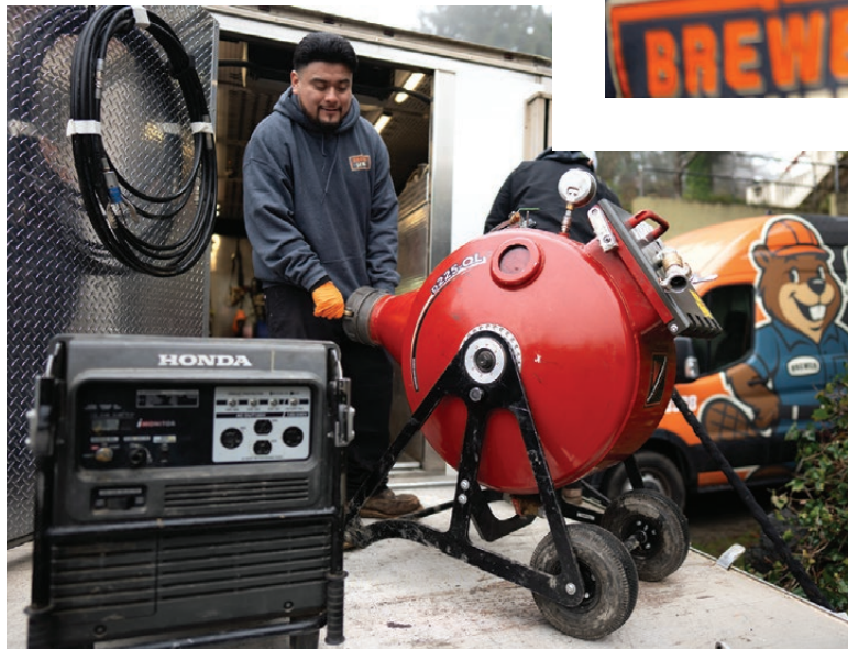
▲ Aldo Morales and Miguel Perez-Sanchez prepare a HammerHead Bluelight system for a liner installation.
