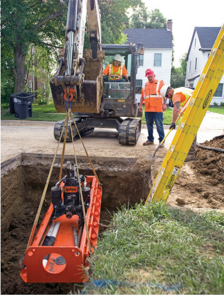
« Connor Goecke uses a Bobcat E60 to move a Roddie Pit Shot horizontal drill into place as Josh May and Logan Pontis look on.
